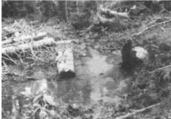
Above, improper location is the principal cause of trail problems. Trail bike volunteers quickly eliminated this situation with 150 feet of relocated trail. Below, problems solved: the relocated trail on stable ground.
