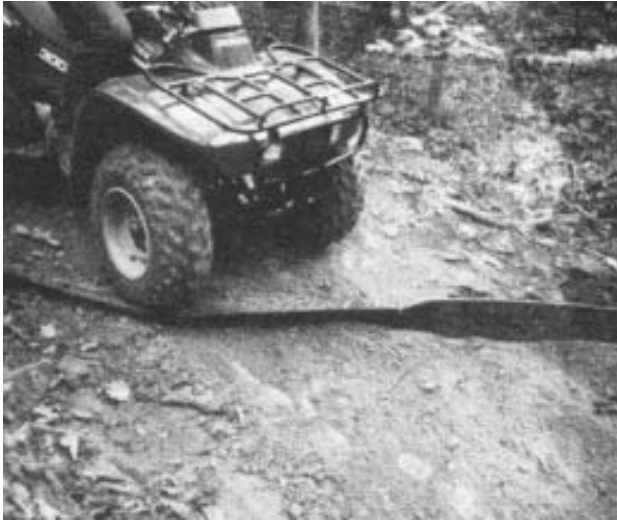
An All-Terrain Vehicle crosses a flexible water bar. Note how the belting allows passage with no changes in terrain to the rider.
