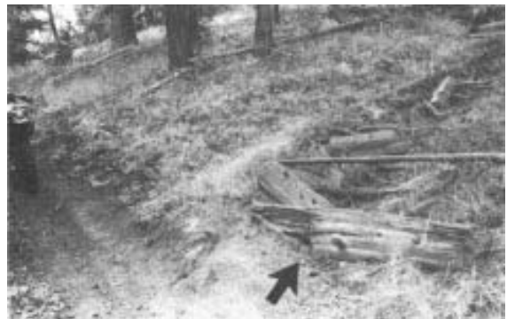
Abandoned trails can be easily and effectively closed by filling with logs and brush.
