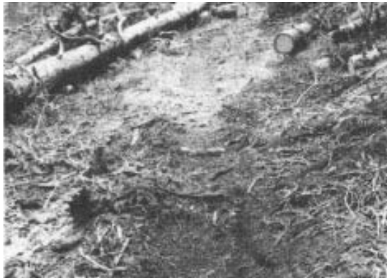
Above, improper location is the principal cause of trail problems. Trail bike volunteers quickly eliminated this situation with 150 feet of relocated trail. Below, problems solved: the relocated trail on stable ground.
