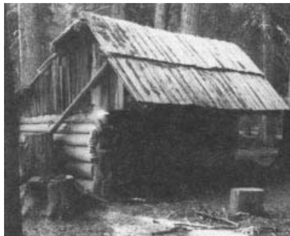
Shelters such as the one pictured above maintain the rustic appearance of the trail while providing an excellent facility for a rest site or camping area.
