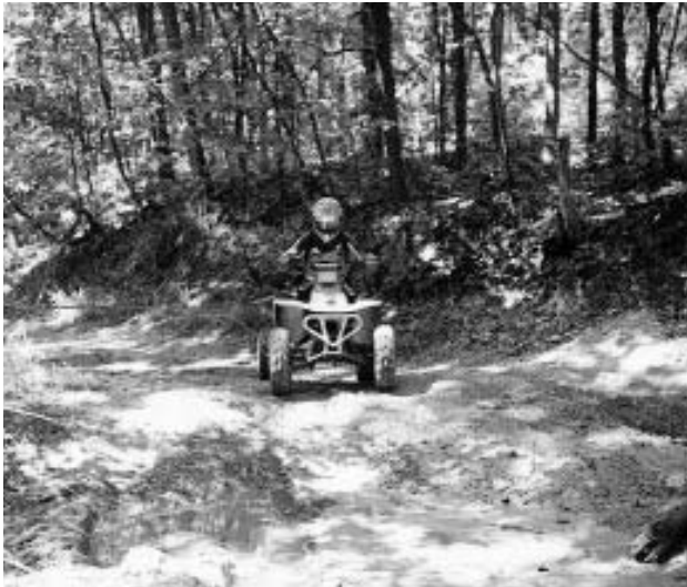
This water-saturated trail tread indicates improper location, improper design or both. This trail should have had an interceptor ditch located 10 feet uphill (See interceptor ditches).
