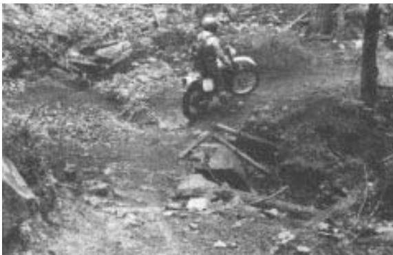
This well-designed stream crossing with its rock bed and sloped approaches reduces impacts while allowing for easy travel.
